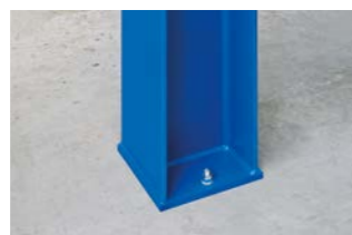
Rigid portal structures allow small pillar bases, which are secured using dowels.
